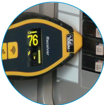
Finding Breakers or Fuses
